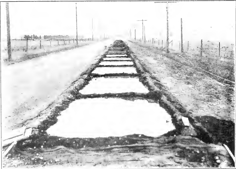
10' Concrete Pavement, Highway No. 27—Curing Pavement by Ponding.
